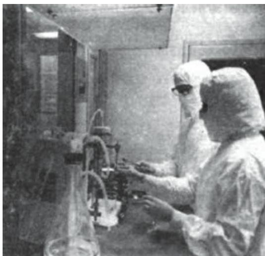
**Fig. 23.9:** Aseptic filling of vials with liquid under vertical laminar airflow, followed by stoppering with forceps by hand
