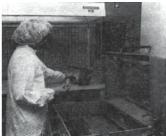
**Fig. 23.7:** Rinser designed to clean vials by racks sized to shipping cartons or by individual handling. Note laminar airflow to protect clean, wet vials
